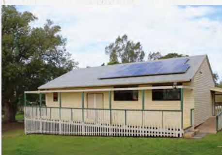
Scout Hall entrance and verandah
